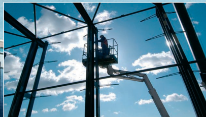
Steel frame assembly
