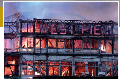
Fire damage in 2003
