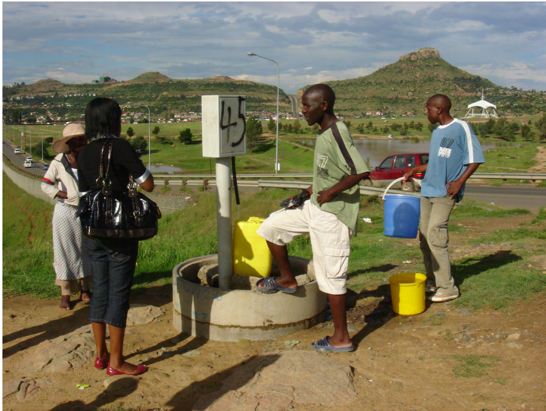
Picture 2: People drawing water from a prepaid system in Ha Thetsane
