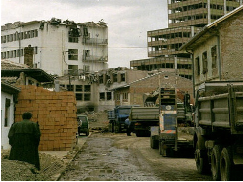
A communications and bank building in Kosovo, destroyed during the fighting.
