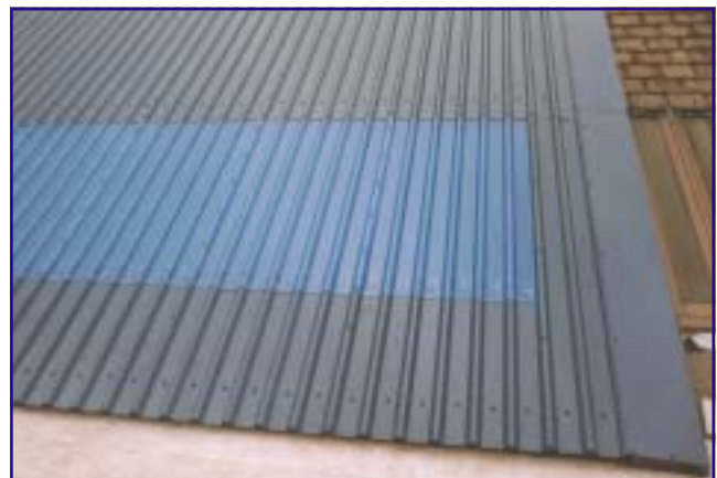
Fig.2 - FILON SupasaFe Blue Tint Fitted to Metal Profile, Underlap and Overlap, Illustrating Good Profile Matching
