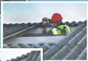
4. Installing fixings
