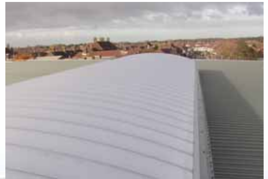
Top: Six barrel vaults on these premises in Sussex were replaced with Sun Modul Finesse units which were fixed directly to the existing upstands. Above: Sun Modul Finesse units were installed by Valent Roofing on this standing seam roof project in the North of England.
