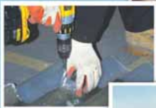
3. Drilling Fixsafe sheet, using old sheet as template
