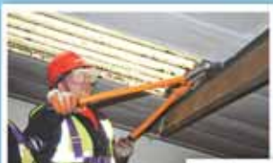
1. Removing hook bolts
