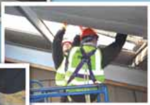
2. Extracting existing sheet
