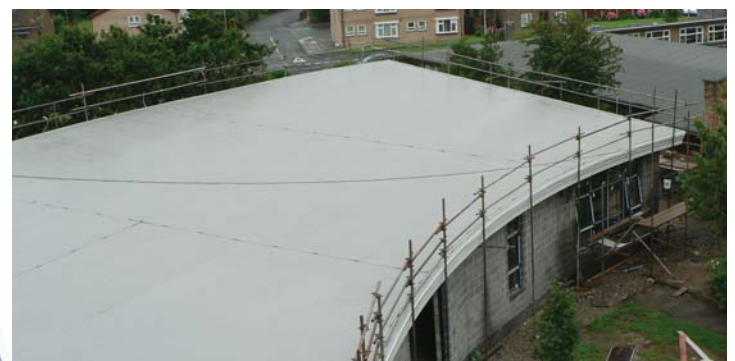
The roof at Mereside Primary School under construction
