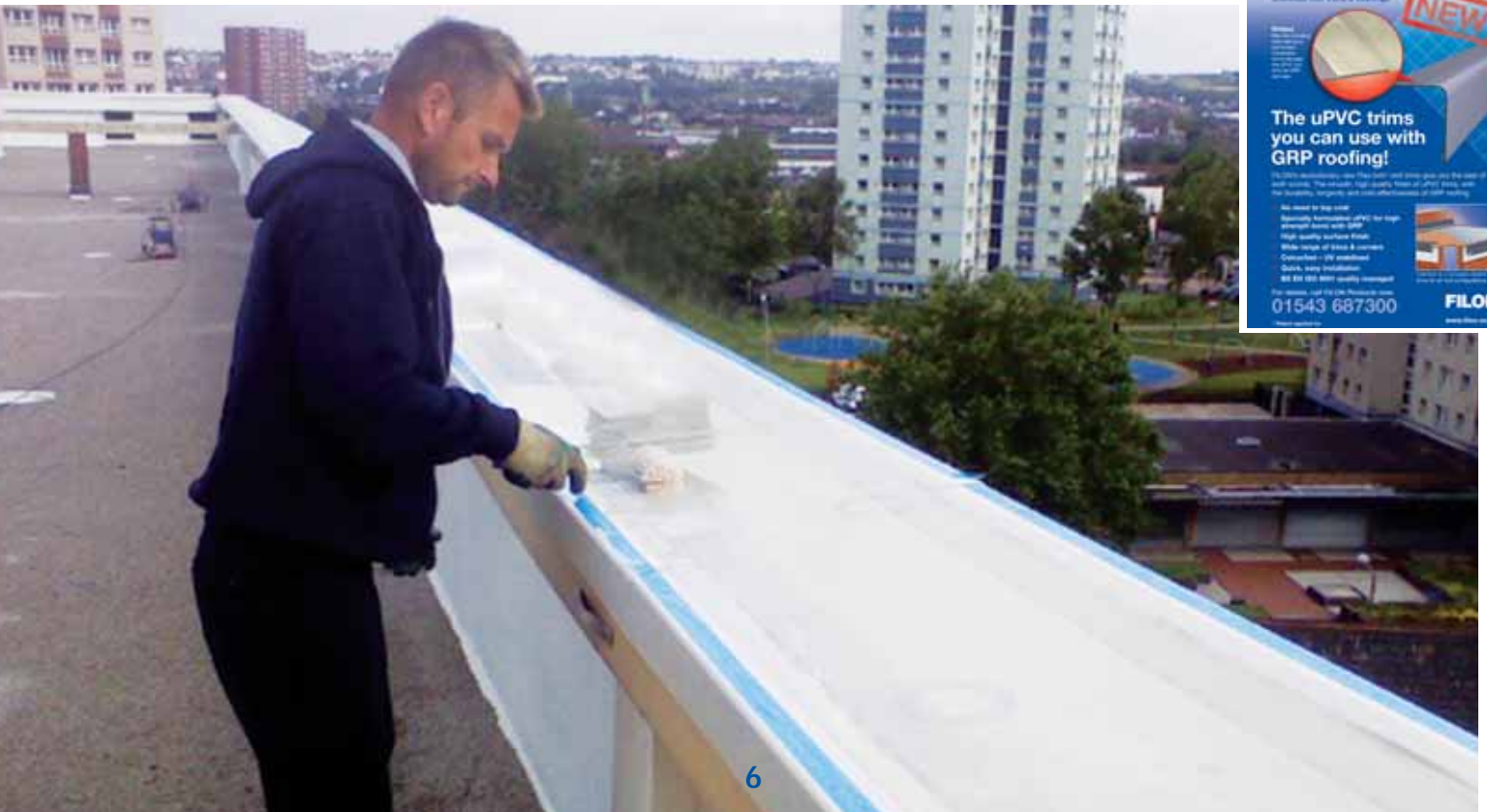
Flextrim installation, Bristol.
