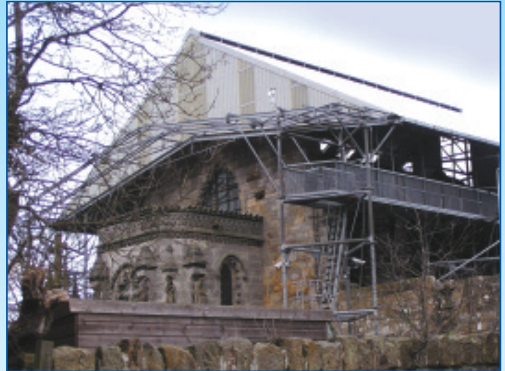
Protective structure for restoration at Rosslyn Chapel, featuring FILON rooflights
