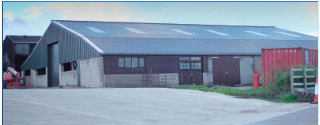
FILON over-roofing, with Profix spacer & insulation
