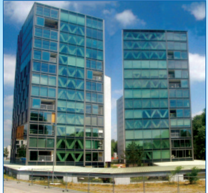
The Chasse Park Apartments in The Netherlands with the car park shown below
