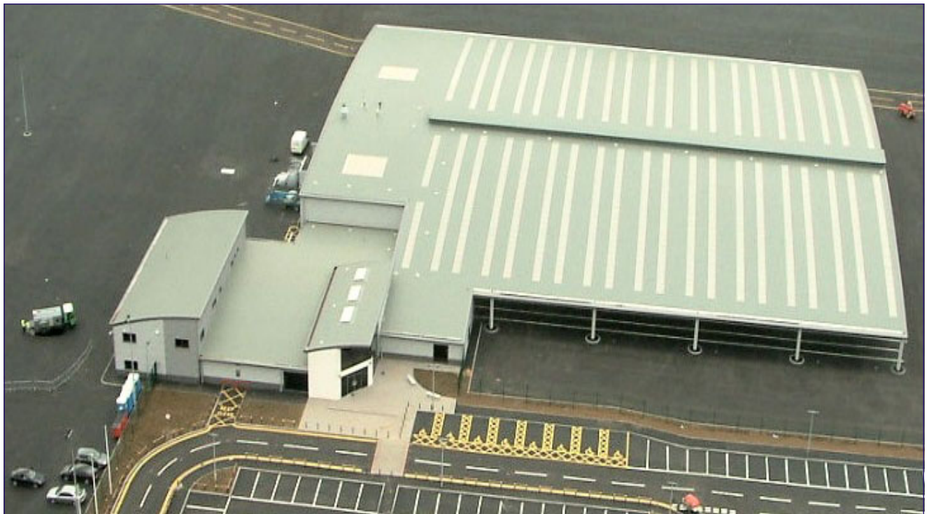
FILON Rooflights used on British Car Auction Building in Bedford
