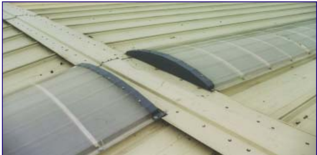
FILON MONARCH Ridge Down Application which Illustrates the Moulded GRP Stop-Ends.
