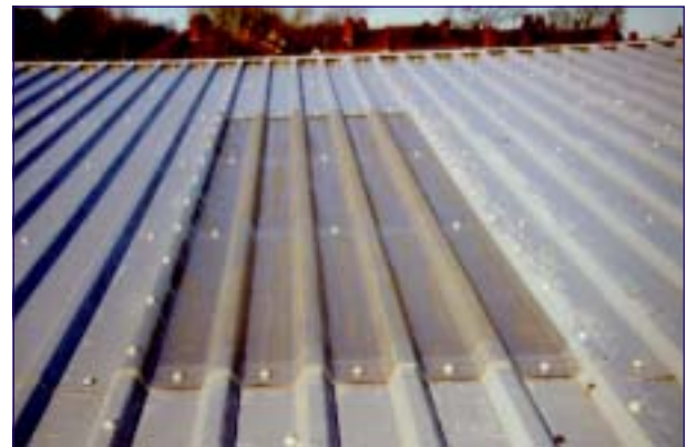
FILON SupasaFe Fitting to EP 32/1000 Illustrating the Good Profile Definition
