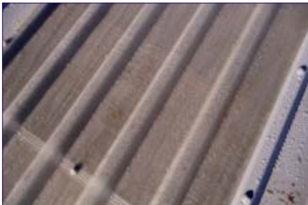
FILON SupasaFe Showing the Stitched Glass Mat Reinforcement
