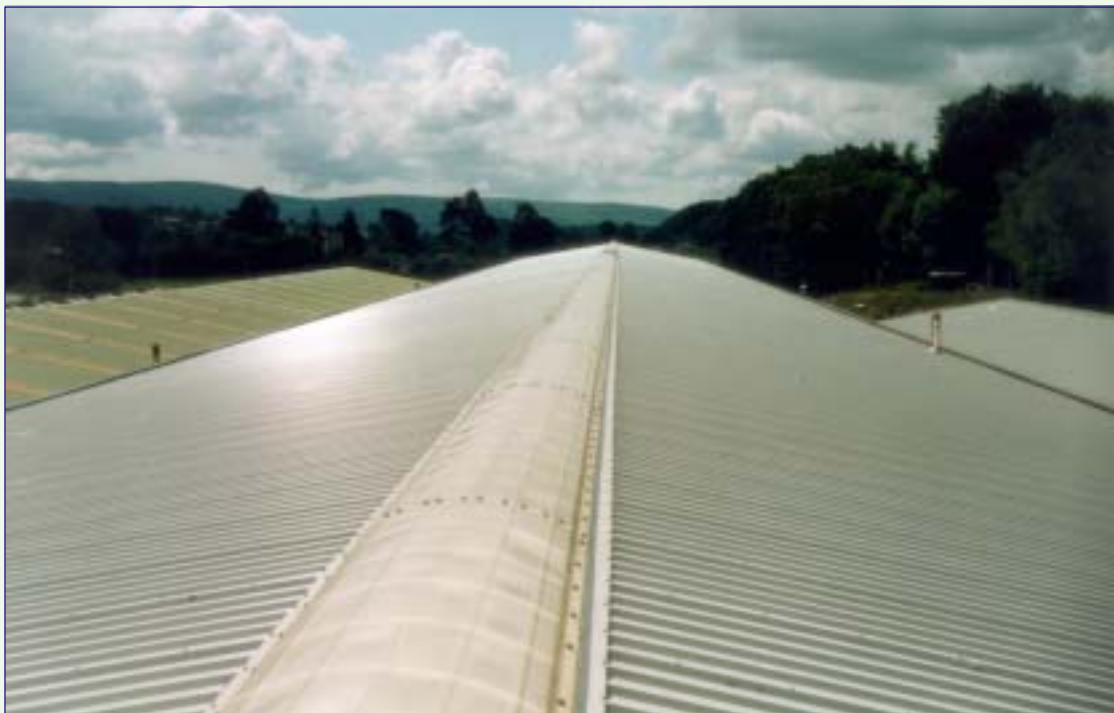
Typical FILON Monarch Application at the Ridge
