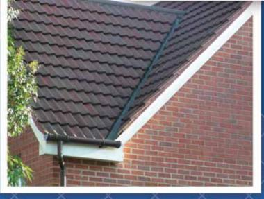
V-Flow valley gutters can be used with all kinds of tiles and slates, as well as profiled roofing systems.
