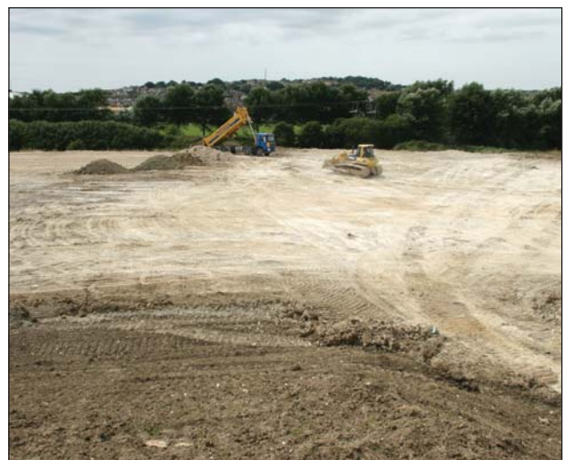
Landraising at Eastside Business Park
