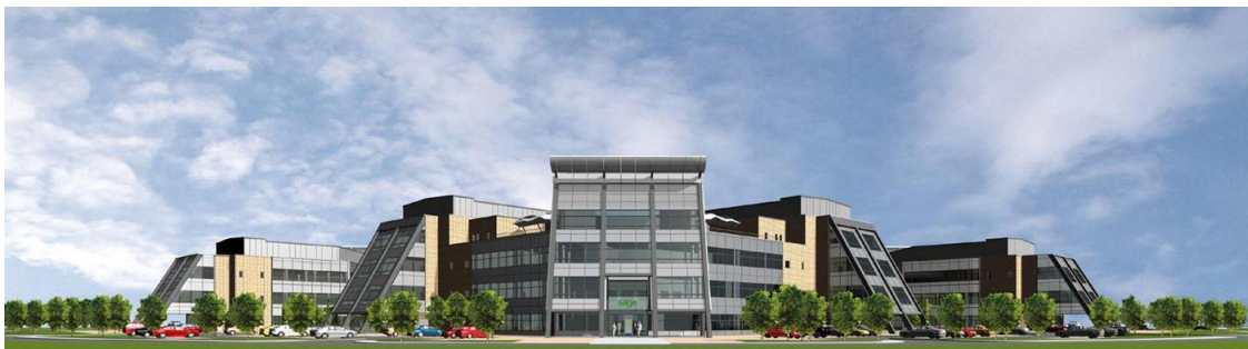
Sage Group plc headquarters, Newcastle
