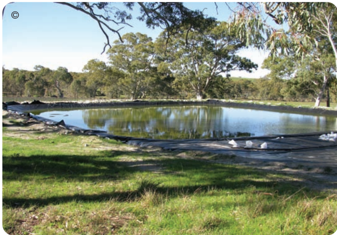
Dam before cover installed
