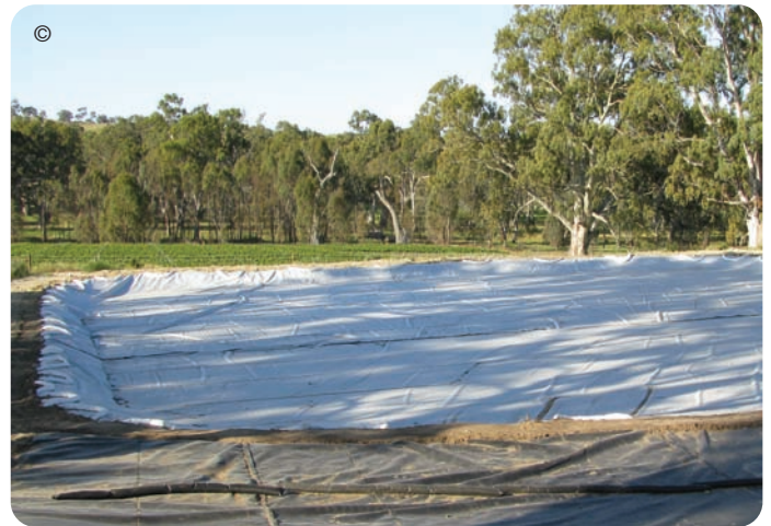
VapourGuard cover installed by Fabtech
